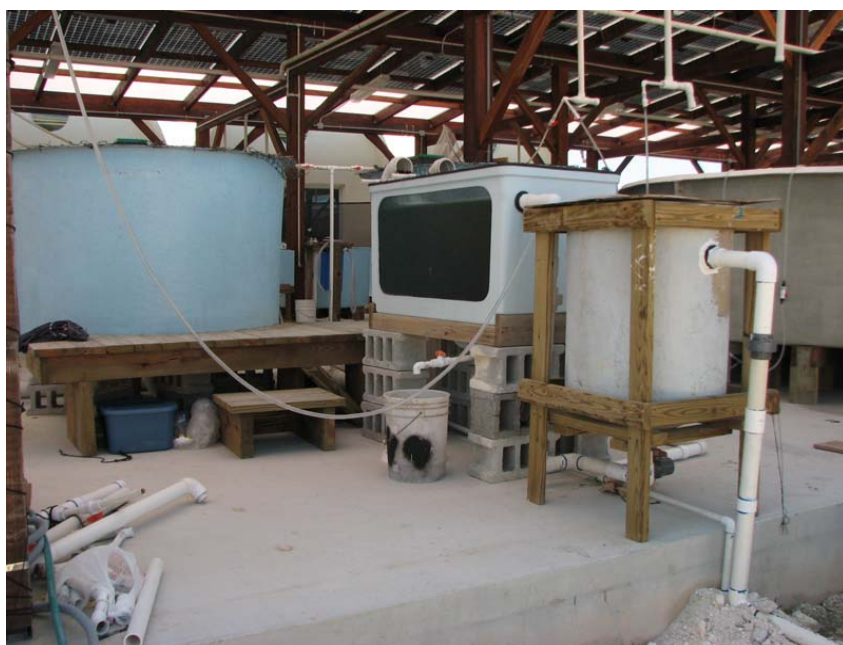
The Tilapia fish tanks, the settlement tank, and the biofilter are all housed in the Wege Center for Sustainable Fisheries – the world's first solar-powered hatchery and wet lab center.
